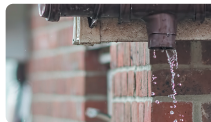
Broken or blocked guttering
